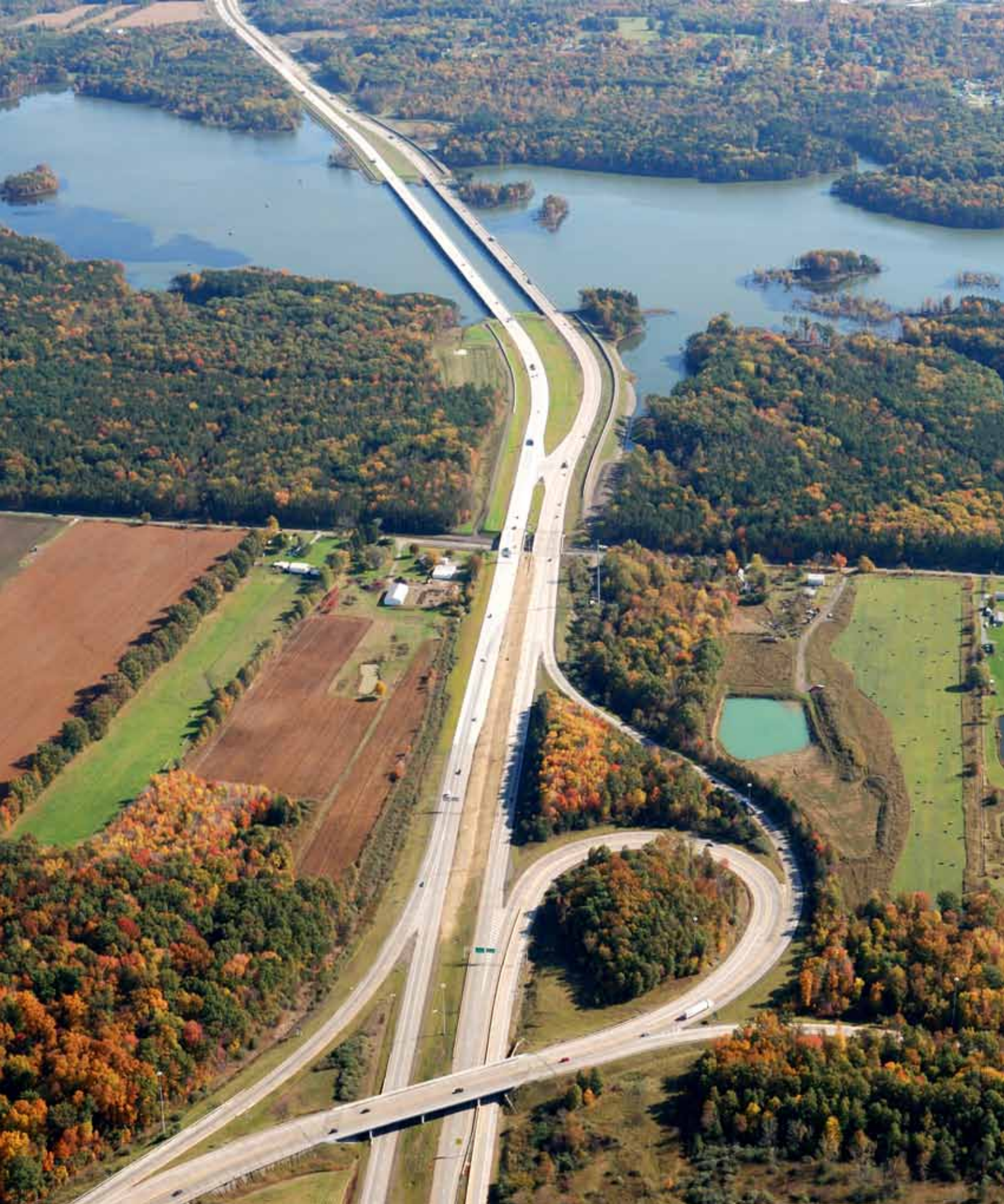
First Place: "I-80 Widening & Bridge Replacement at Meander Reservoir"
