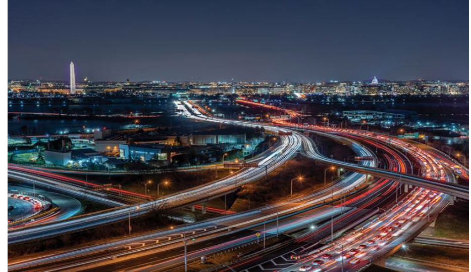
Photo Source: FHWA .
