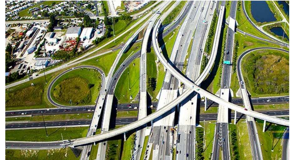
Photo Source: FHWA .
