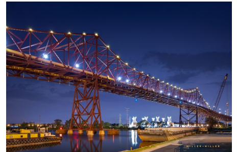
Operations of the Chicago Skyway Toll Bridge were awarded as a P3 lease concession in 2004.
