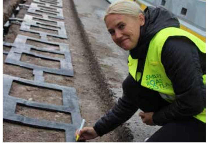
Laying road segments. Image courtesy of Electreon.
