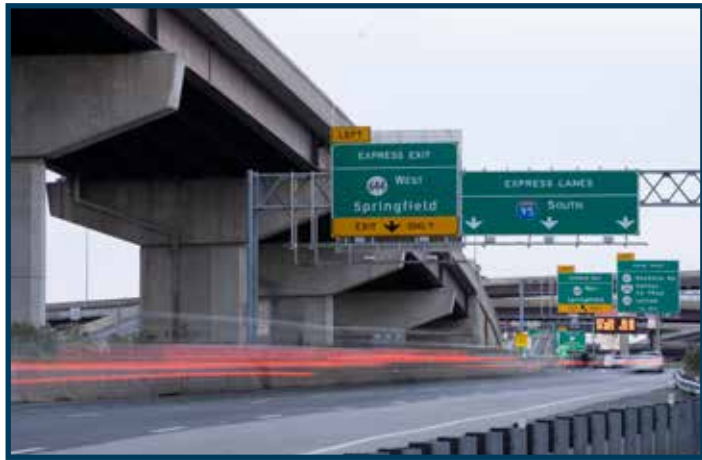
The I-95 Express Lanes in Virginia run northbound in the mornings and southbound in the evenings. Photo courtesy of Transurban.
