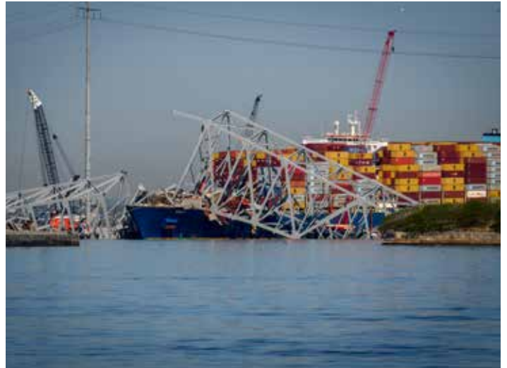
The collapsed Francis Scott Key Bridge rests on top of the cargo ship Dali in the Baltimore Harbor in an undated photo provided by MDOT.
